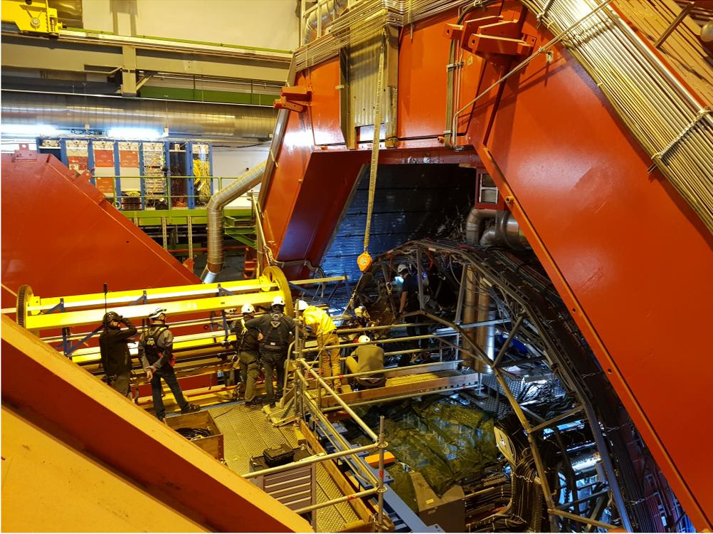
Figure 8.11: The TRD supermodule 6 was removed after we had uncabled it.
