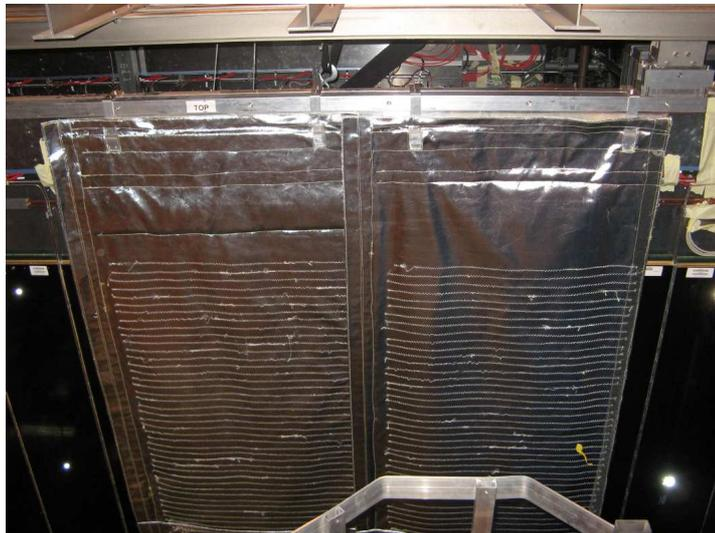
Figure 16: Installation of the heating blanket in Point 8.
