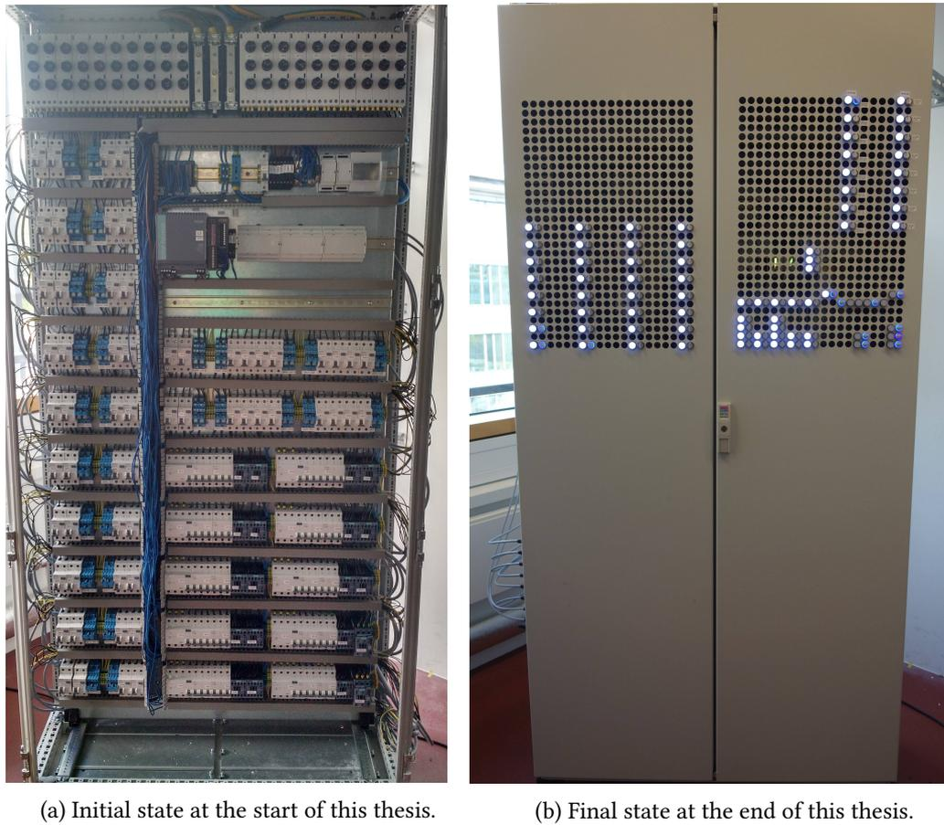
Figure 32: Power control unit for the GI-HAS experiment. Initial state (a) was built in *Paknejad (2017)*. Addition of outer shell, connection to main power supply, integration of control hardware and override switches, set up of input sensors, and programming of control logic was done to arrive at the finished power control unit (b).
