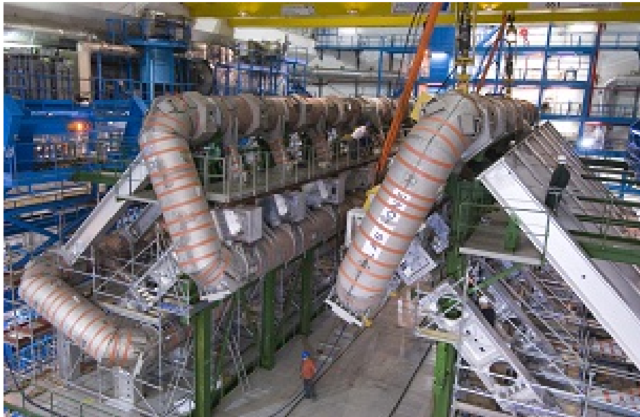
Figure 2.8: The ATLAS toroidal magnet system in its construction phase. (Image from [5])
