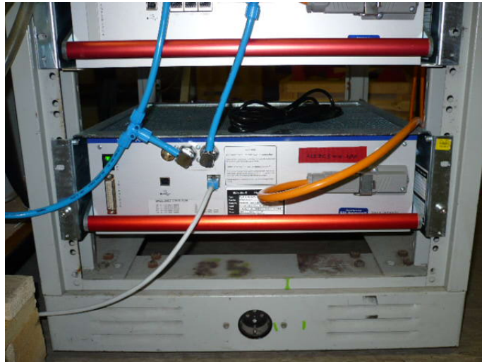
Figure 3.5: A Wiener Power Supply mounted in a crate at the lab at Heidelberg. The two blue tubes provide water cooling. The gray Ethernet cable keeps it under remote surveillance. The orange cable provides 220V to the power supply.
