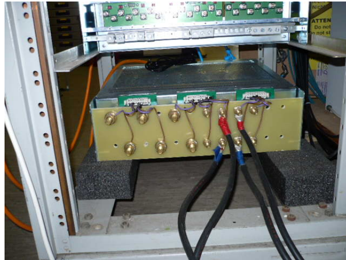
Figure 3.6: Backpanel of a Wiener power supply. In total there are 8 available channels with two are used in the test setup at the Physikalisches Institut in Heidelberg. One channel is for the power control unit (left) and one for the power distribution box (right). The cables are marked with blue for ground and red for power.
